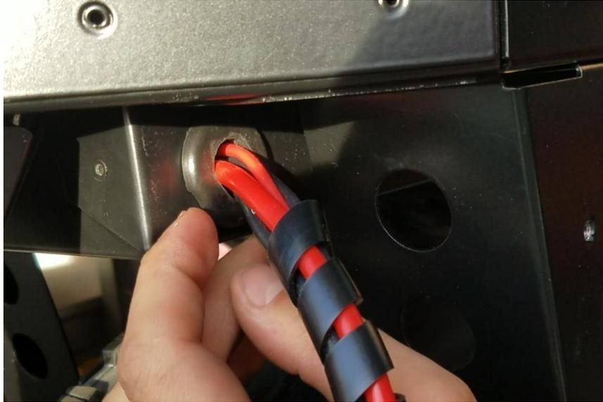
11. Push at least one inch of the cable wrapped harness into the battery compartment.
